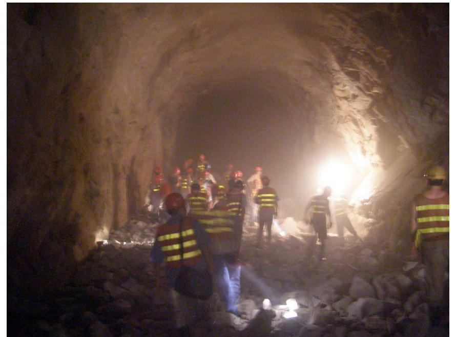
Main Tunnels Join - June 09
