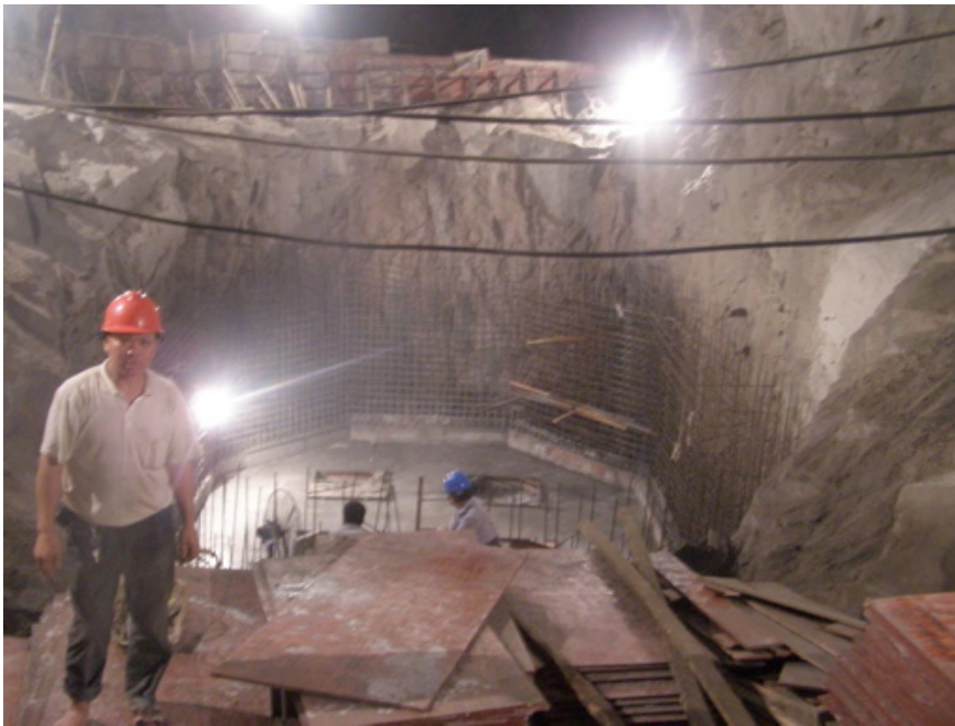
Pool Excavation in DBY Hall - Aug 09
