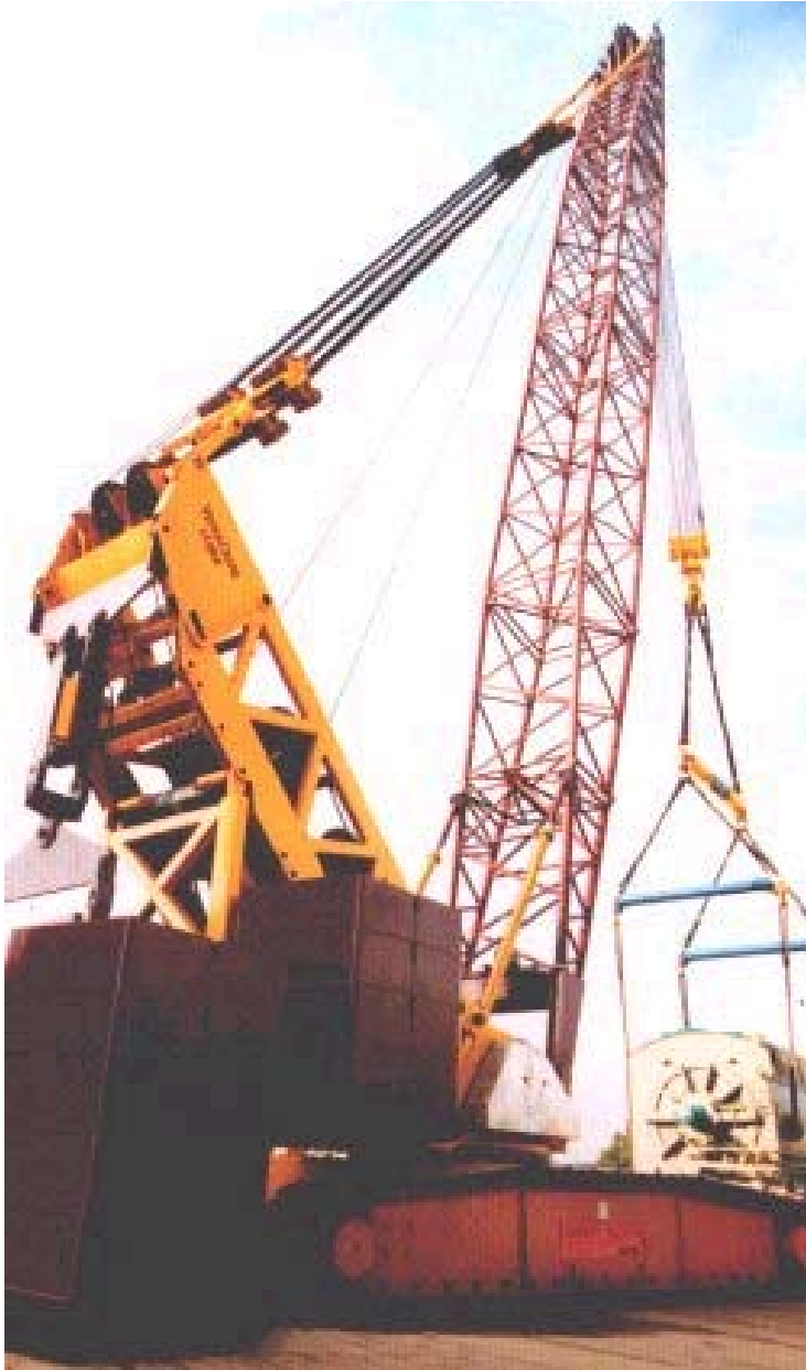
Transporting 550 ton Coker Drum from ship to crane hook
