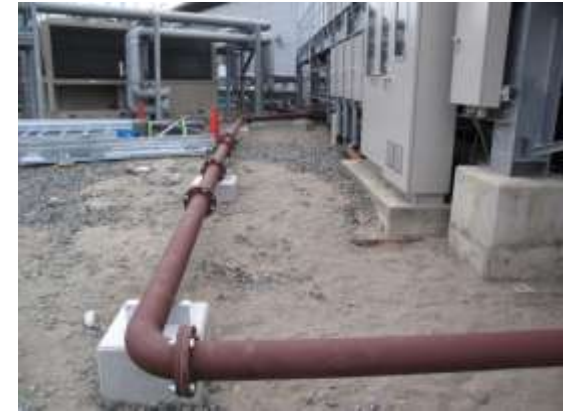
Water pipes were replaced, being ready for passing water.
