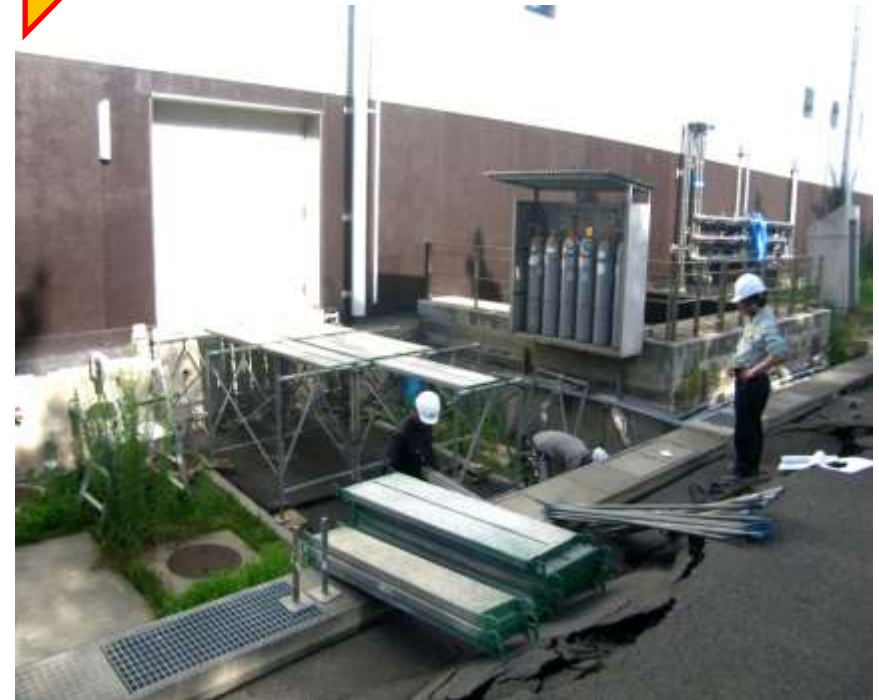
Placing a temporal bridge for carrying in materials for repair.
