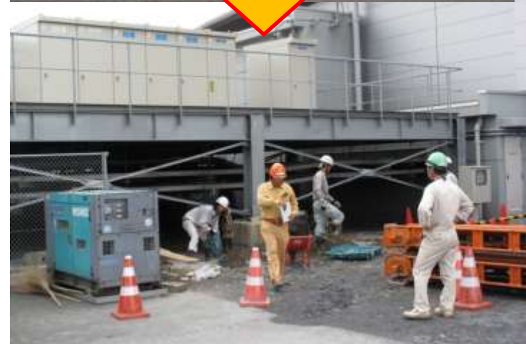
The bent stage was repaired. Power has been supplied to the RCS building.
