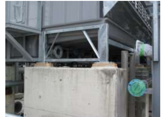
Reinforced foundation for a cooling tower (right) Refining work of pumps and motors (left)
