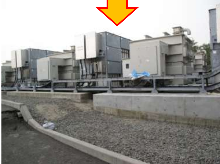
Tilted condenser transformers were straightened.
