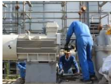
Reinforced foundation for a cooling tower (right) Refining work of pumps and motors (left)
