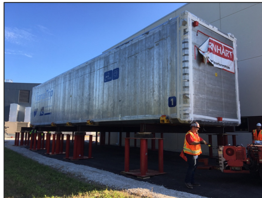
Behind the ICARUS building – July 26
